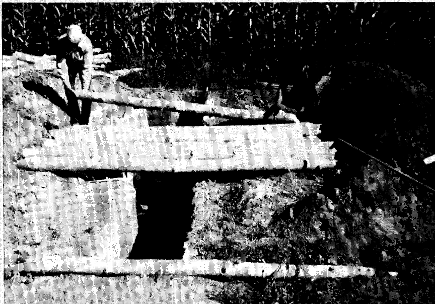
Placing 9-foot poles for the roof of a Pole-Covered Trench Shelter.
