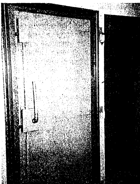
Steel door leading into "Faraday Cage" which houses FEMA-Region IV communications room at Thomasville, Georgia.
