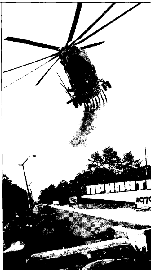
Helicopter decontamination in progress near Chernobyl reactor site.
