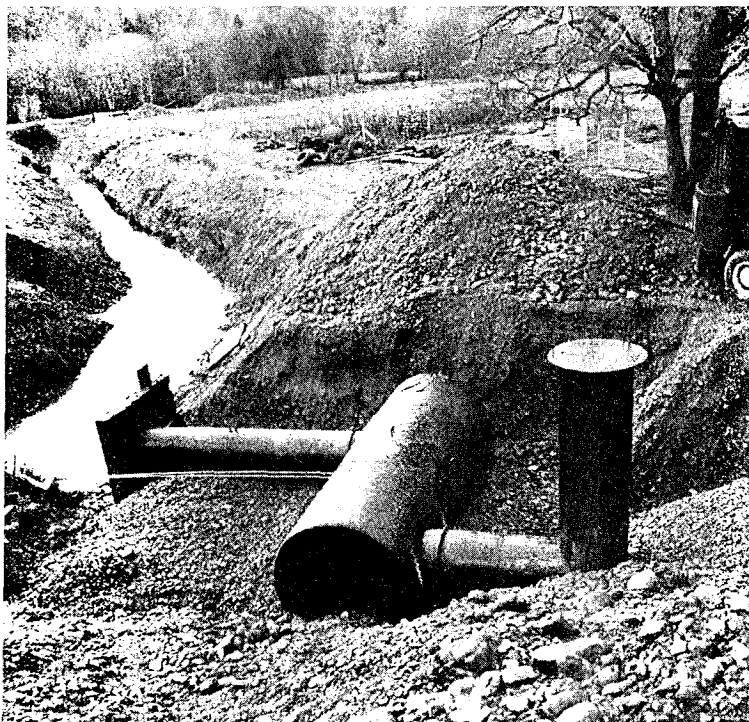
Metal blast shelter in place on Robinson ranch ready for finishing touches and backfilling.
