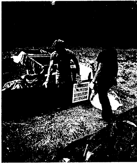
OISM man and wife volunteers at work on above-ground door-covered fallout shelter with earth roll walls — from NWSS.
