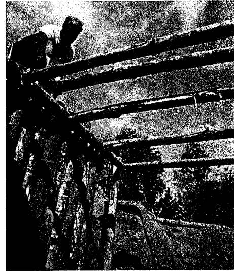
OISM volunteer at work on small pole blast shelter — from NWSS.
