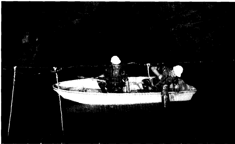
Left: Technicians check out one of the mountain's reservoirs — 400 feet long, 15 to 18 feet deep and V-shaped to absorb nuclear shock waves.
