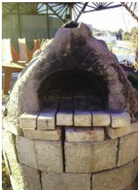
Earth type oven-can be used for several days with the heat remaining in the oven.
