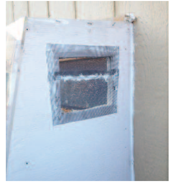
Vent on upper side
