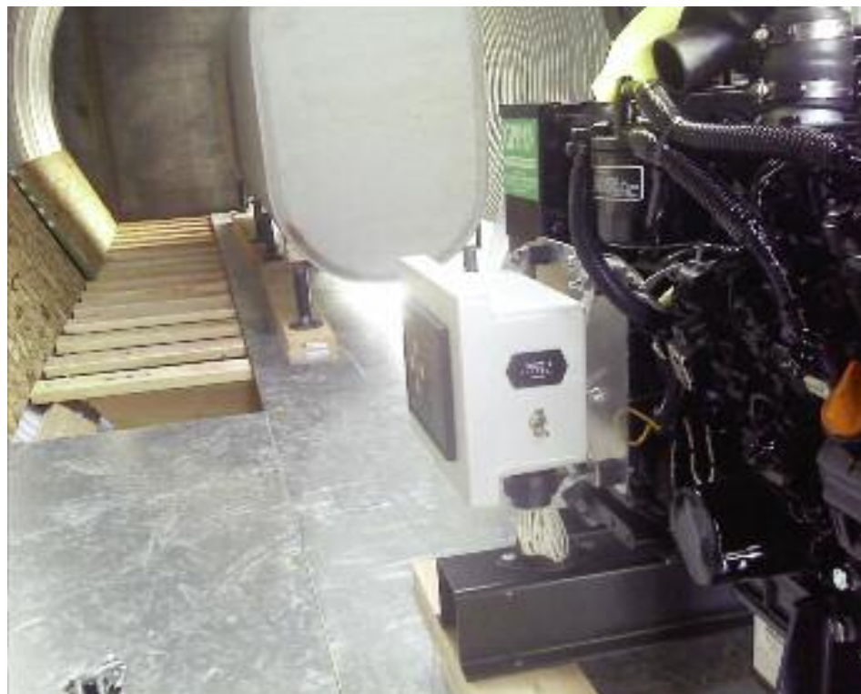
We keep redundant solar charge controllers, inverters, chargers and DC breakers (for each shelter), inside faraday cages for use after an EMP.
