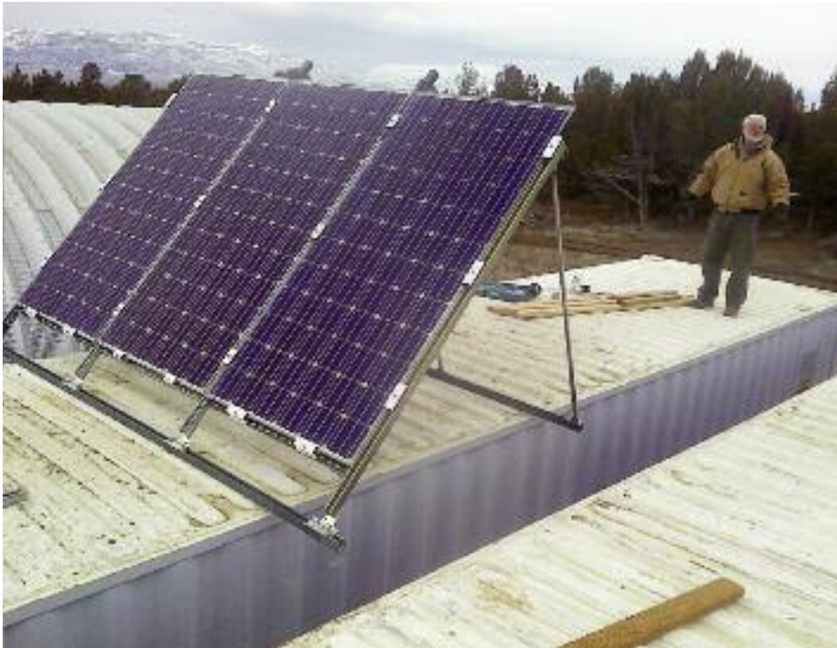
We have placed three, 300-watt solar panels in frames on top of the storage unit. We have frames ready for five more panels (which are currently stored and EMP protected inside our steel shelters), but will not place them outside until well after an attack.
