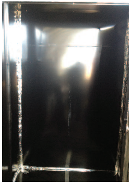
Sealing Seams Inside of Steel Cabinet with Aluminum Tape
