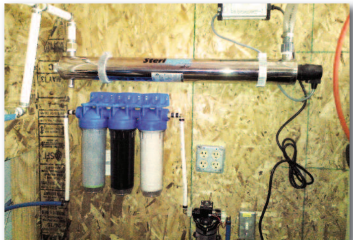
2. Large Sterilight UV sterilizer disinfects up to 8 gallons per minute.
