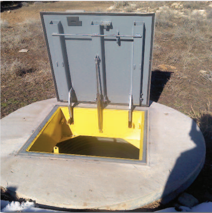
Typical shelter access hatch. Provides security and shelter integrity.
