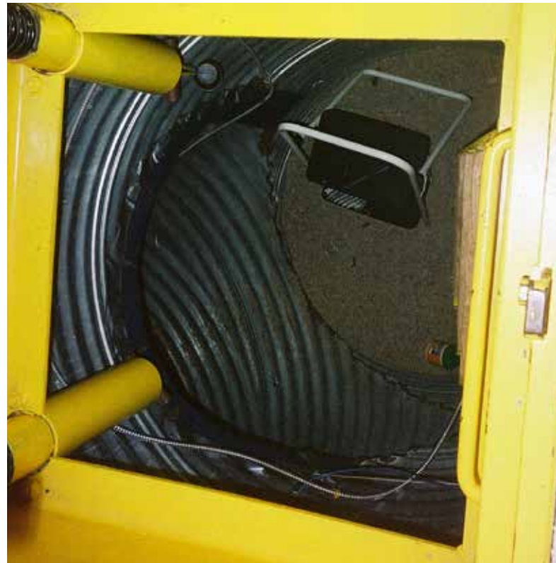
Figure 3 Ladder to Entrance
